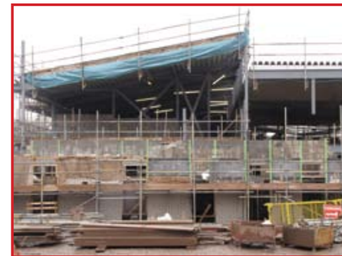
St Anne's under construction
